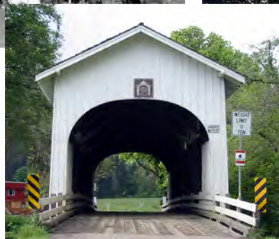
Harris Covered Bridge
